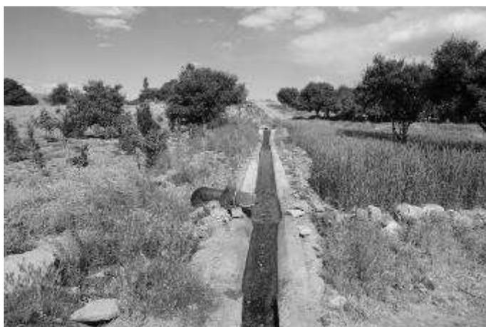
Figure 2.2. A view of the traditional irrigation water supply by cemented canals
