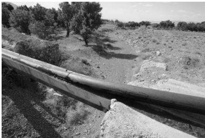
Figure 2.7. Using existing canal for support of the pipeline instead of building a bridge between upper & lower reservoir pool
