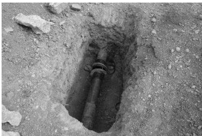
Figure 2.6. The Broken part of the pipeline by over passing a tractor machine
