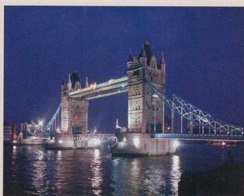
▶ Most Na Tamizie – Tower Bridge
