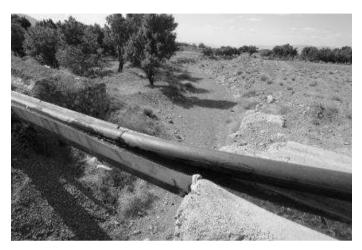
Figure 2.7. Using existing canal for support of the pipeline instead of building a bridge between upper & lower reservoir pool
