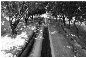
Figure 2.4. New pipeline system beside the old cemented canal
